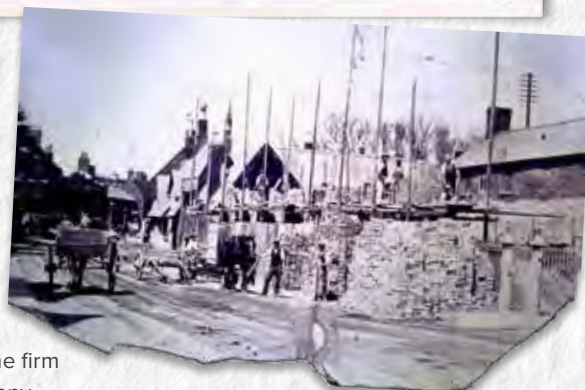
The main building under construction, see book cover
